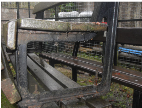
In need of repair!
