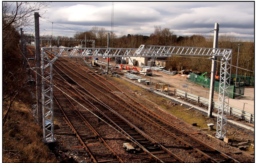
Two new gantries for supporting the overhead wiring, installed just to the south of the road bridge at Oxenholme station.
