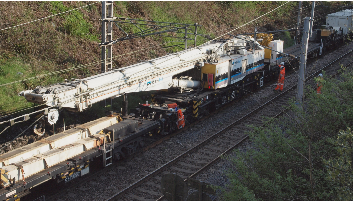
Above: the massive 125t Kirov crane, for lifting track panels into place.
