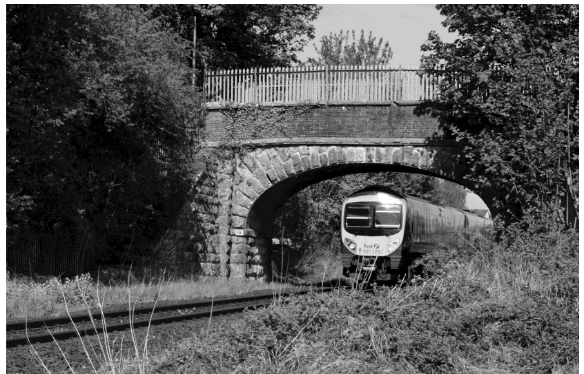
Bridge 16, between Sparrowmire and Briarigg: the parapet will need to be improved, but there is clearance for the overhead wires.
