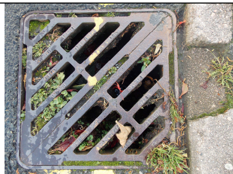
Blocked Drain, Helm Road, Bowness
