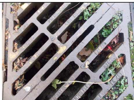
Blocked Drain, Helm Road, Bowness
