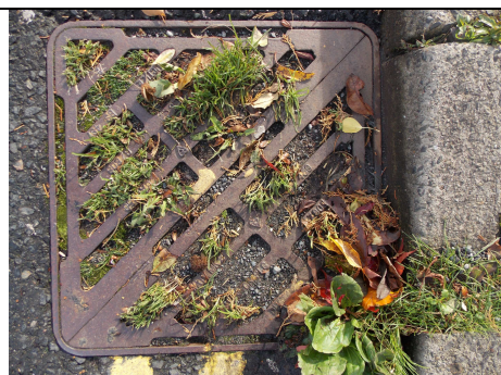
Blocked Drain, Helm Road, Bowness
