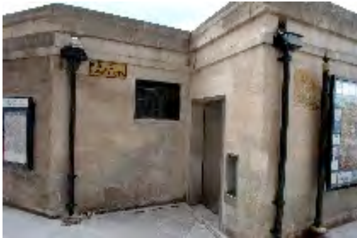
Bath and North East Somerset Council's superloo is clad in local stone to meet with Bath's strict planning laws
