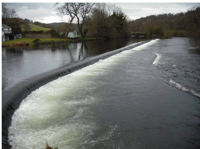
Newby Bridge weir with flood sluice on left bank.
