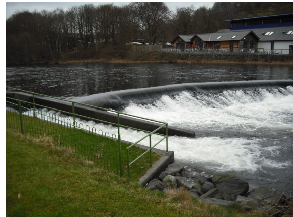
Ainsworth Dam looking towards left bank with fish pass visible on the left of the photo
