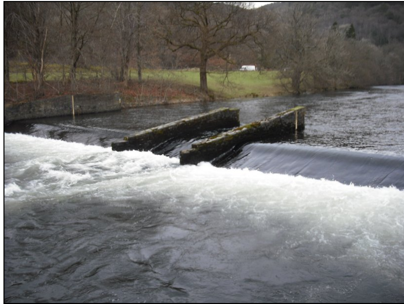
Figure 4.3 Newby Bridge Gauging Station Compound Weir
